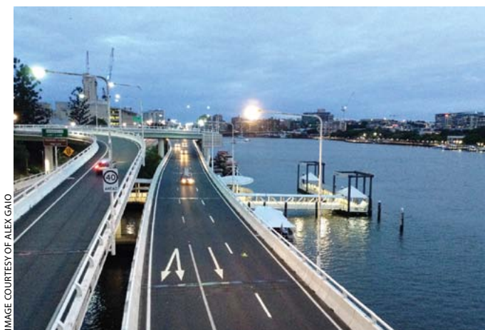
Riverside Expressway in Brisbane. Here, it's stacked on top of the Riverwalk
